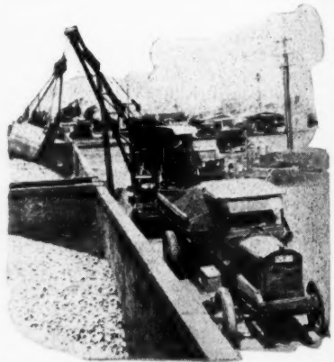
The Universal Unloading on the Job.
